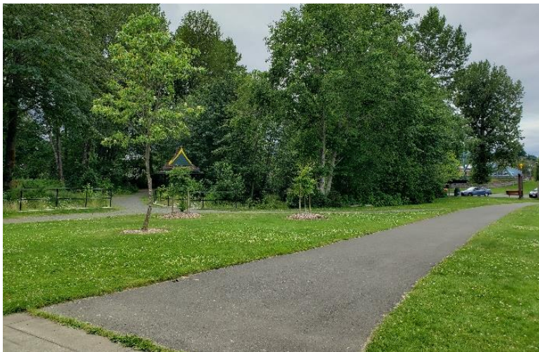
Figure 21: Arrow #3 looking west near existing culvert
