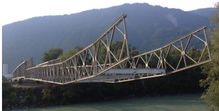
Figure 36: Truss being push-launched with launching nose attached
