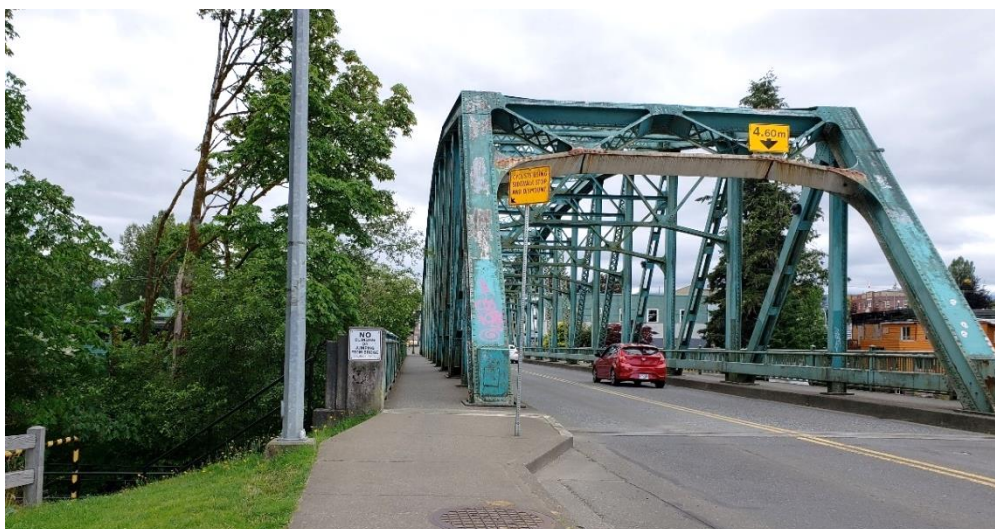
Figure 2: View west of the existing 5 th Street Bridge sidewalk
