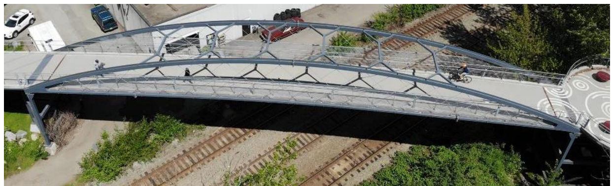
Figure 40: Harbourside West Pedestrian Bridge in North Vancouver, BC
