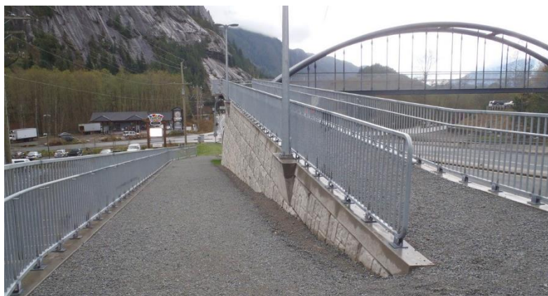
Figure 14: Example of standard Ministry bicycle fence in pedestrian bridge application
