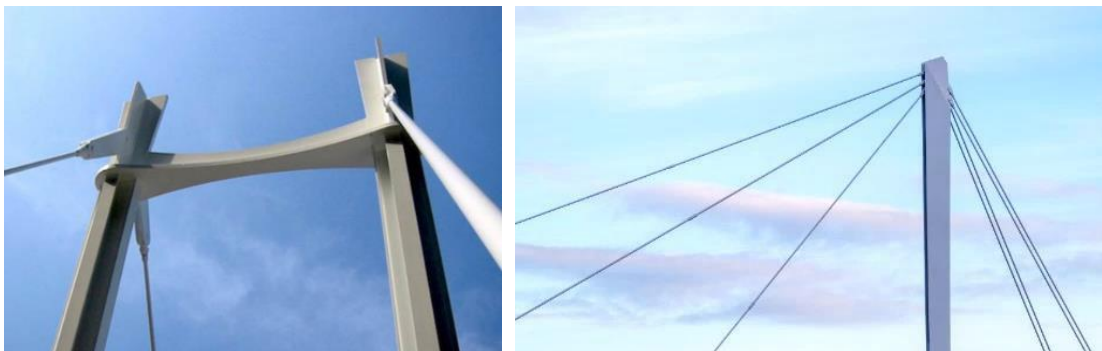
Figure 47: Examples of sculptural steel pylons
