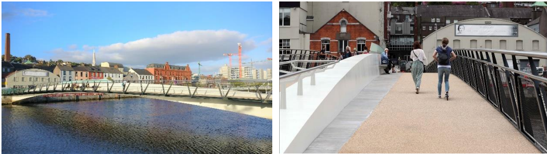
Figure 49: Mary Elmes Pedestrian Bridge in Cork, IR is an example of a raised torsion girder span
