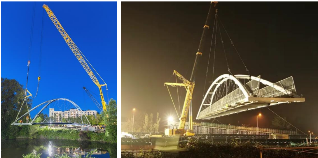
Figure 41: Examples of arch pedestrian bridge lifts
