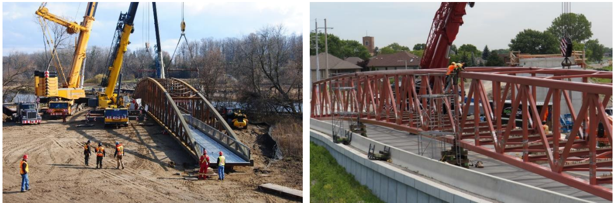
Figure 29: Construction of pre-engineered truss pedestrian bridges – Walter Bean Trail Bridge in Kitchener, ON (left) and Cousineau Pedestrian Bridge in Windsor, ON (right)
