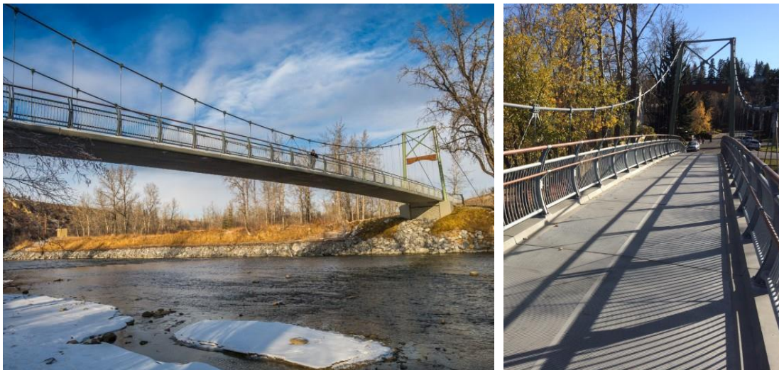
Figure 50: Elbow River Suspension Pedestrian Bridge in Calgary, AB.
