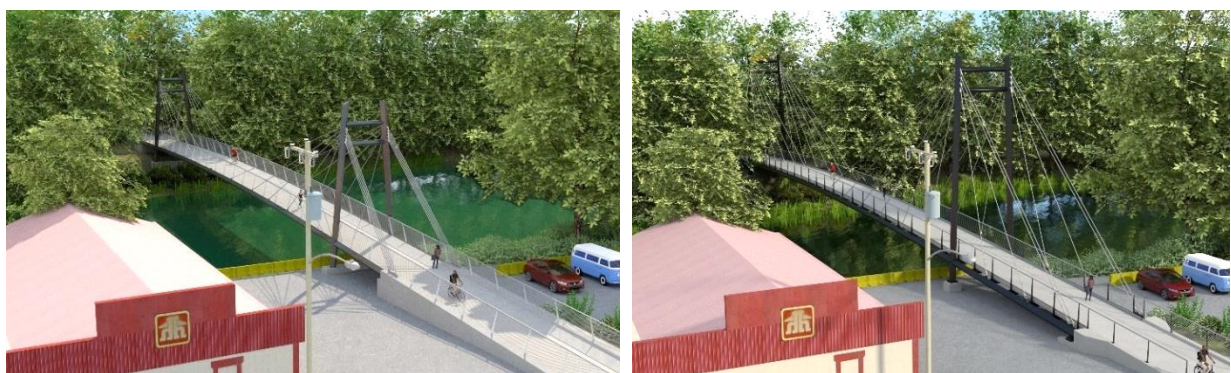
Figure 44: Renderings of cable-stayed bridge option with shorter (left) and taller towers (right)
