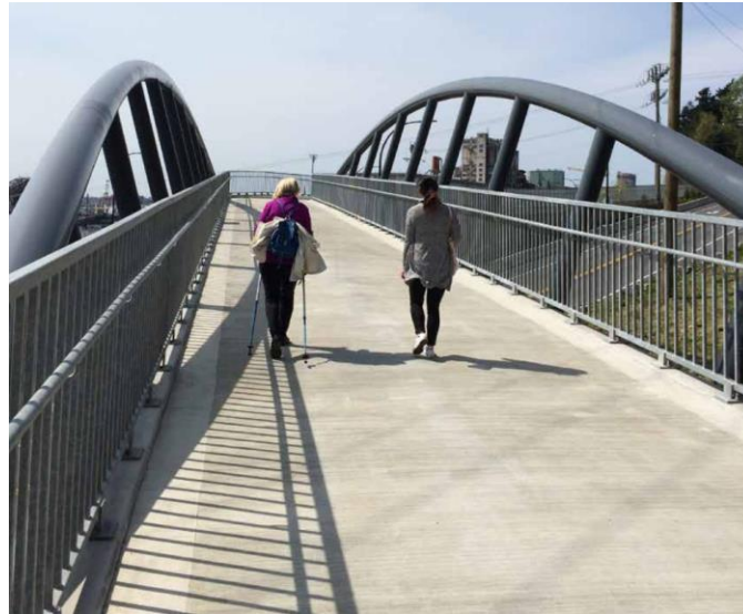
Figure 12: Example of concrete deck surface on a Spirit Trail pedestrian bridge
