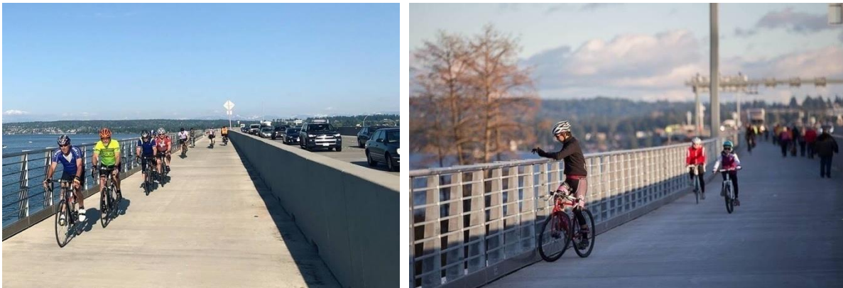
Figure 51: mixed-use 4.26m wide pathway on SR 520 floating bridge in Seattle
