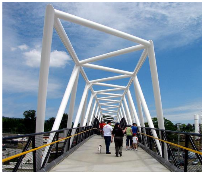
Figure 13: Four-metre wide deck on Central Valley Greenway pedestrian bridge
