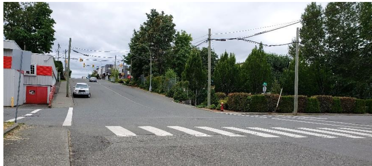
Figure 34: Intersection of 6 th St and Anderton Ave, roadway sloping up to the west
