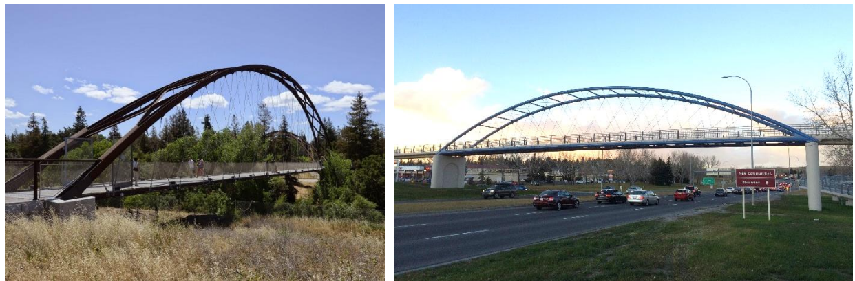
Figure 39: Happy Hollow Bridge in San Jose, CA (left) and Shaganappi Trail Bridge in Calgary, AB (right)
