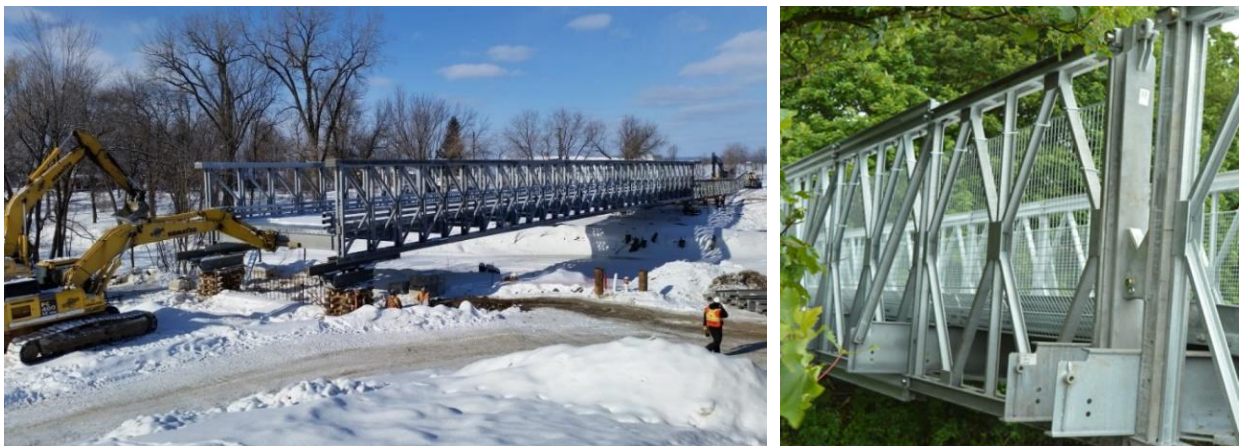
Figure 32: Example of modular panel bridge
