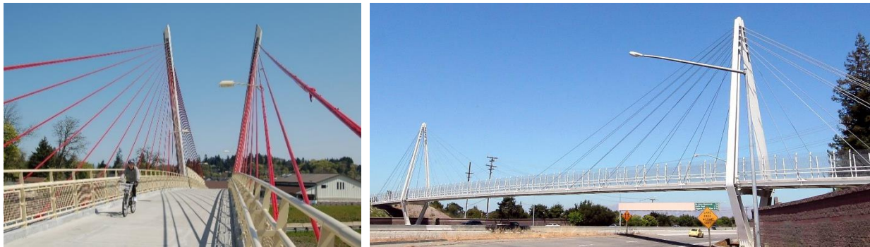
Figure 46: Delta Ponds Bridge in Eugene, OR (left) and Mary Ave Pedestrian Bridge in Cupertino, CA (right)
