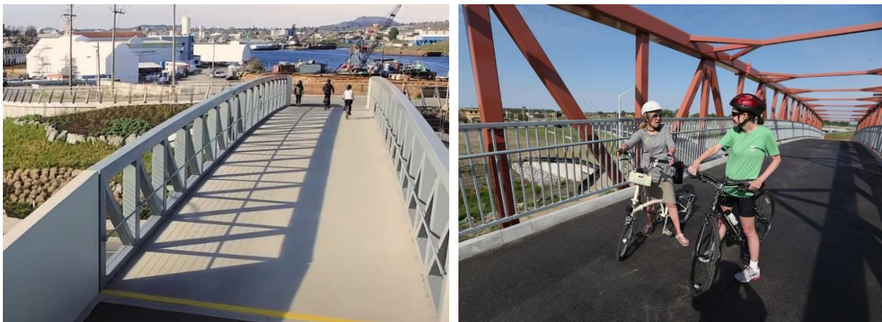
Figure 28: Johnson St Pedestrian Bridge in Victoria, BC with 35m span x 5m wide deck (left) and Cousineau Pedestrian Bridge in Windsor, ON with 60m span x 4m wide deck that uses overhead bracing (right)
