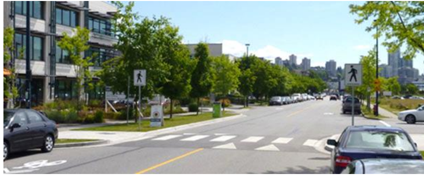
Figure 56: Example of raised crosswalk
