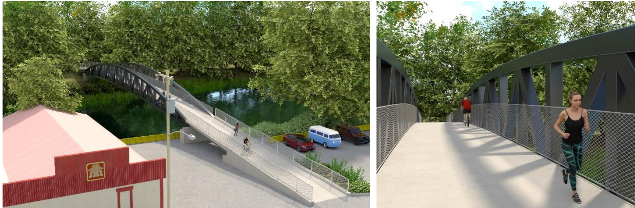
Figure 27: Renderings of pre-engineered bowstring truss option at proposed project location
