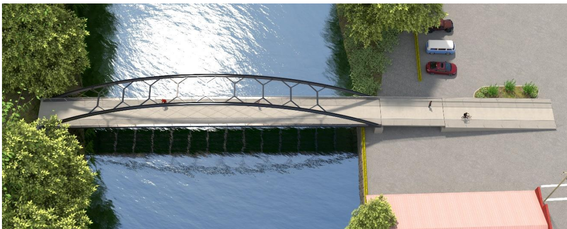
Figure 43: Bird's eye view of network arch bridge option at proposed project location
